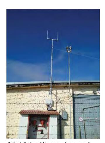
3. Installation of the expander on a wall
