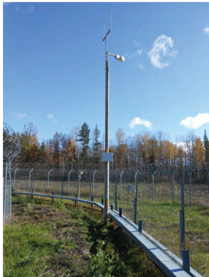
4. Installation of the expander on a lamppost
