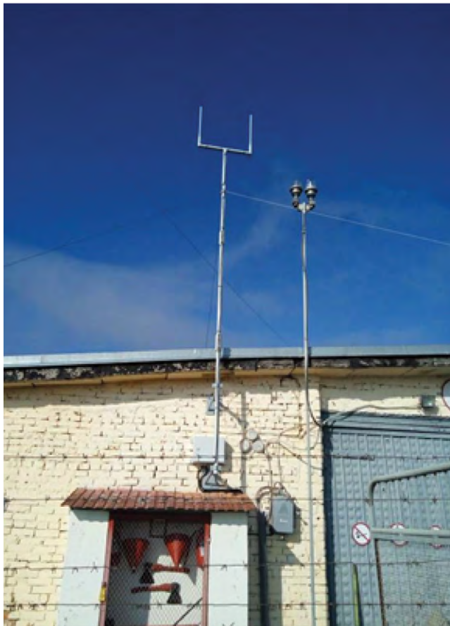
3. Installation of the expander on a wall
