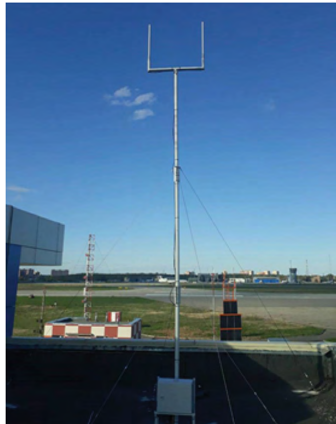
2. Installation of the expander on a roof
